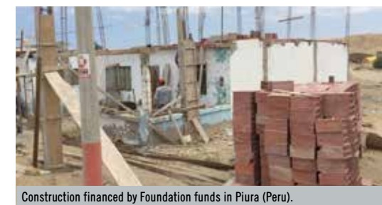
Construction financed by Foundation funds in Piura (Peru).
