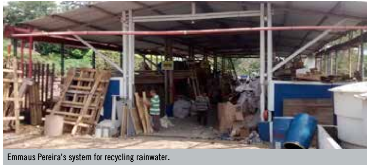
Emmaus Pereira's system for recycling rainwater.
